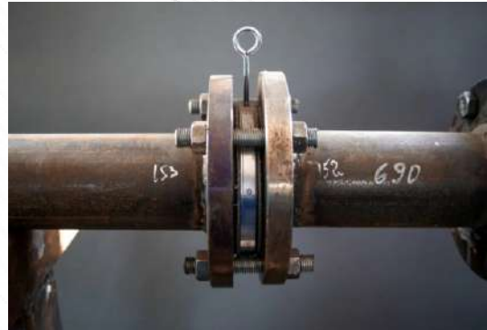
Installation of Flanges
