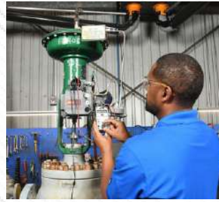
Servicing & Calibration of Control Valves
